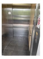
Interior of elevator cab is stainless steel and will require refurbishment or wall panel replacement due to the catering use and delivering of equipment to the ballroom.
